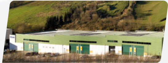
CNC lathes Assembly plant 10,000 m 2 | Mallabia – Spain
