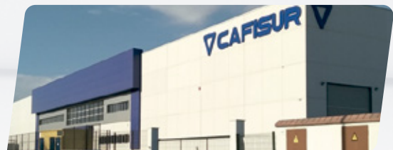
Industrial boiler company 15,000 m 2 | Cádiz – Spain
