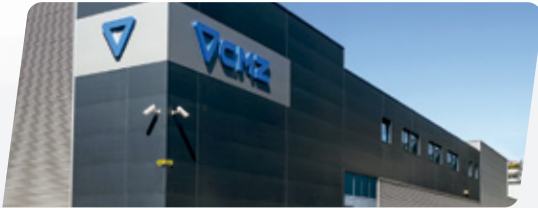
CNC lathes Assembly plant 5,500 m 2 | Zaldibar – Spain
