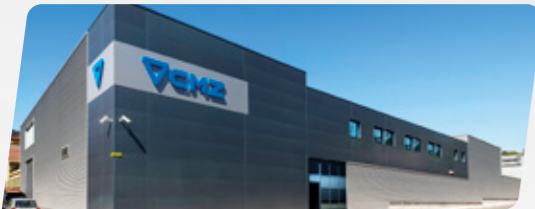
CENTRAL SERVICES | TECHNICAL ASSISTANCE SERVICE Zaldibar – Spain
