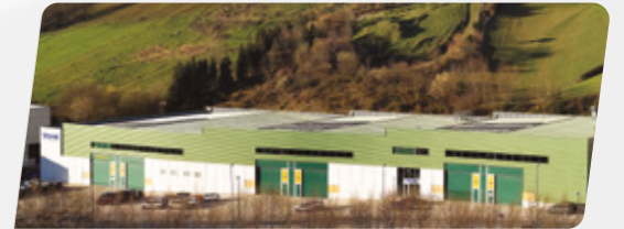
CNC lathes Assembly plant 10,000 m 2 | Mallabia – Spain
