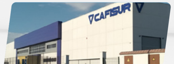
Industrial boiler company 15,000 m 2 | Cádiz – Spain
