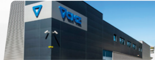
CNC lathes Assembly plant 5,500 m 2 | Zaldibar – Spain
